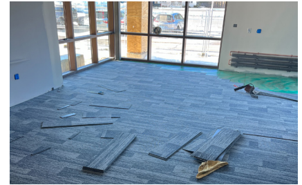
Above: Carpet flooring installation at new addition.
